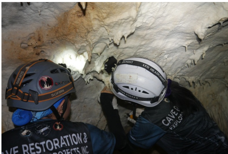
CREP members carrying out repair and restoration work in the B1 section of Five Fingers Cave.
