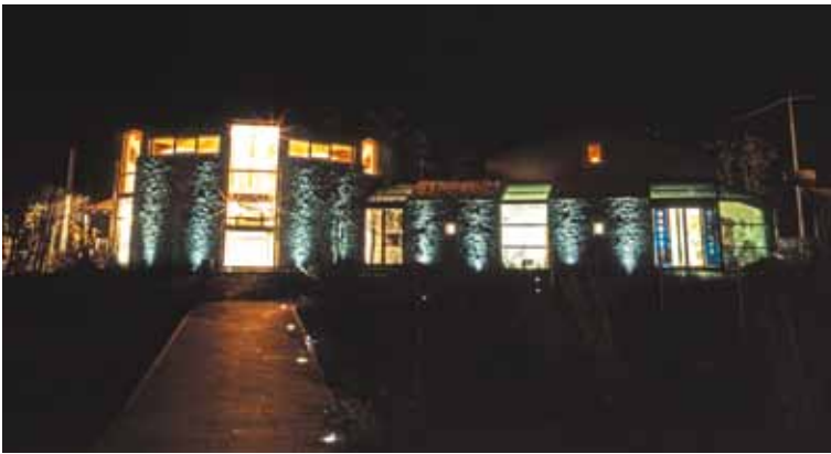
Fig. 2. The new Visitors reception centre of the Grotta Gigante by night. Photo: A. Fabbriatore
