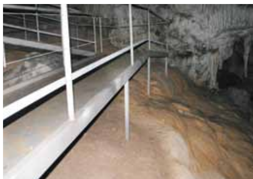
Fig. 4. Method of construction that keeps the cave floor more natural. Archive of Križna jama.
